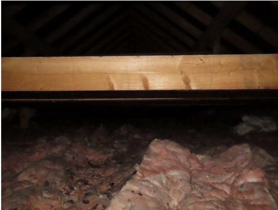
Photo 21 – rat droppings on fibreglass insulation in western attic space
