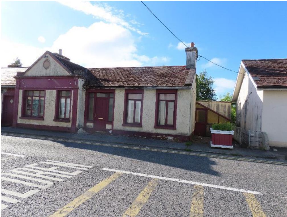
Photo 1 – eastern section of restaurant building with tiled roof – timber fascia missing
